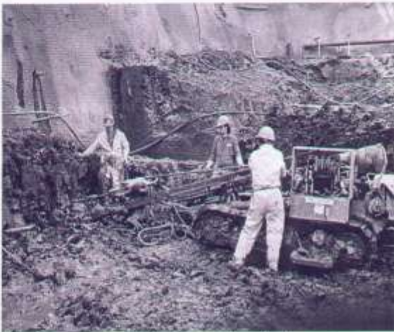
LIKE all GCM jobs, Edmonton shoring was done same time as digging. Space-consuming struts were not needed.
