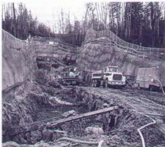
LIKE all GCM jobs, Edmonton shoring was done same time as digging. Space-consuming struts were not needed.
