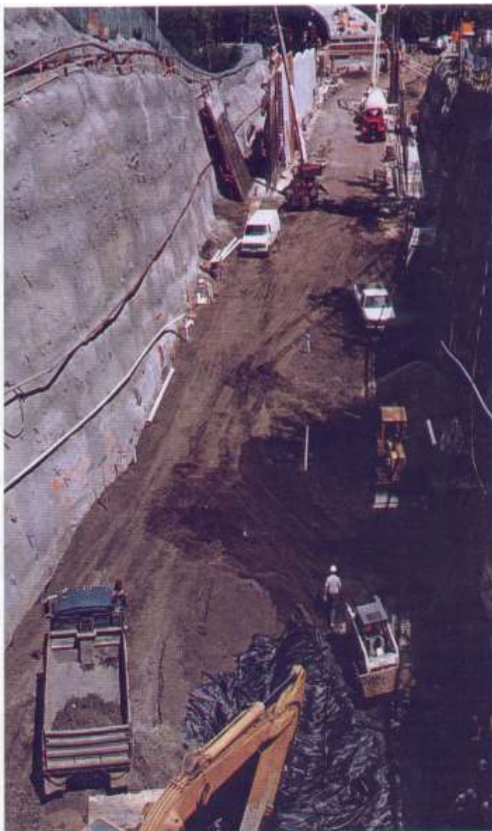
RECORD 20 m deep GCM cut was stabilized for section of Edmonton's LRT system.
